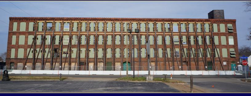
Demolished everything except the brick facade, using specially engineered buttress.
