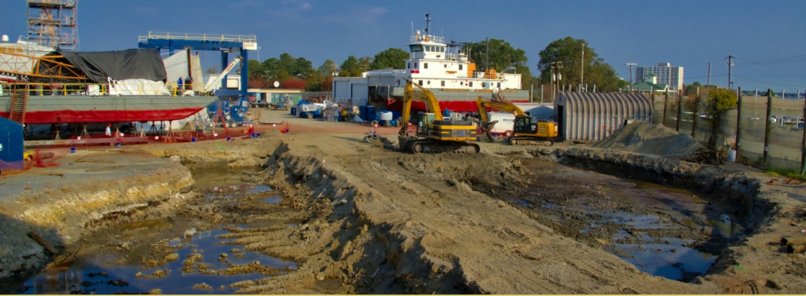
Coordinated and completed in operational shipyard.
