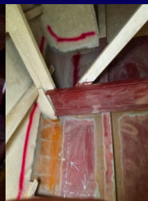
Paint removal for welding pathways enabling hull improvements.
