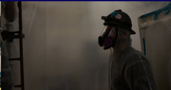
Complete removal of friable asbestos in very tight quarters.
