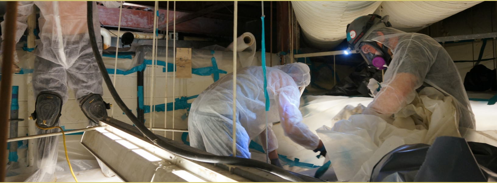
Complete removal of friable asbestos in very tight quarters.
