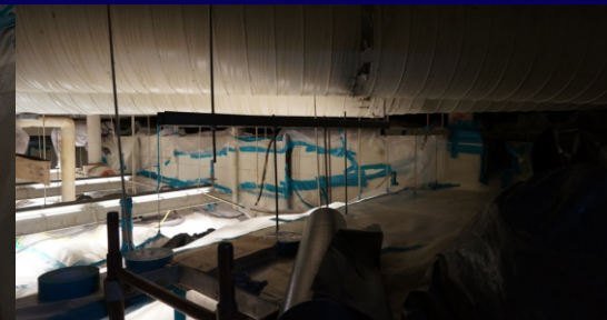
Complete removal of friable asbestos in very tight quarters.
