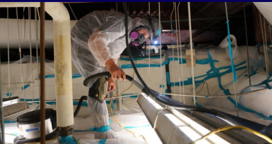
Complete removal of friable asbestos in very tight quarters.
